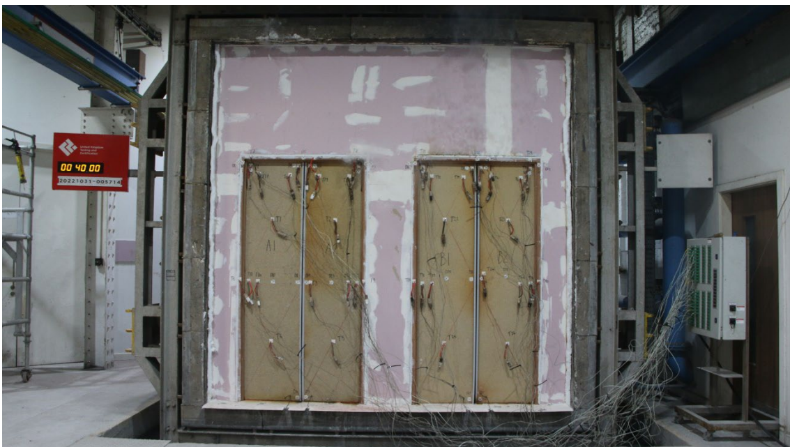
Figure 19 - The unexposed surface of the test construction after a test duration of 40 minutes
