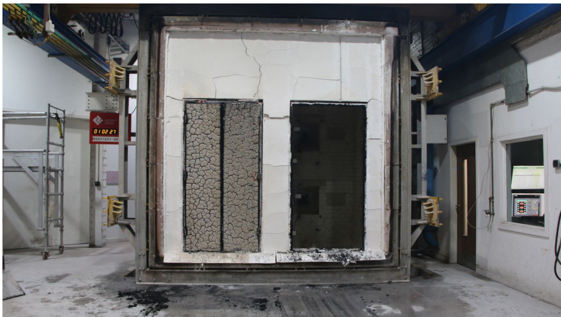
Figure 25 - The exposed surface of the test construction after the test was discontinued
